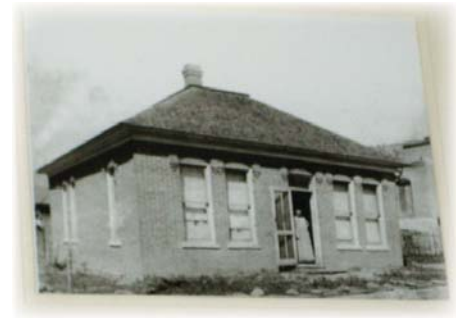
The old and original foundation of the Meadows clinic.
