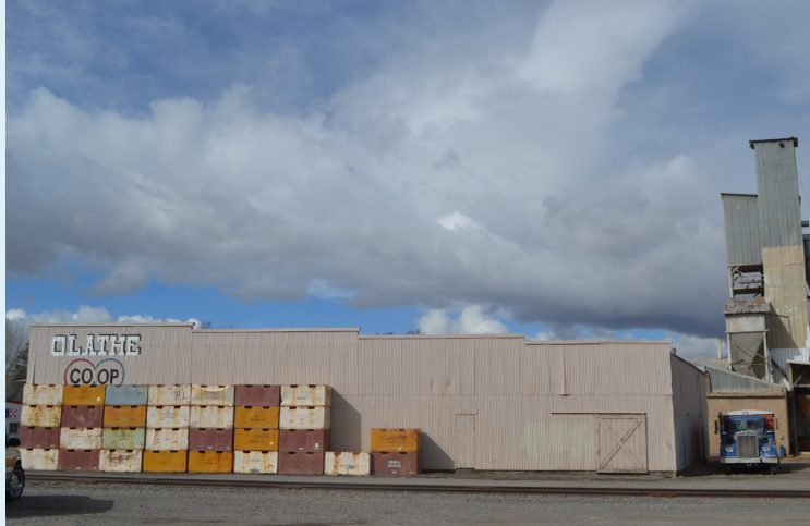
Olathe in Montrose County. Colorado Coalition for the Medically Underserved
